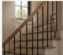
STAIRCASE DETAIL WOOD & IRON BALUSTERS
